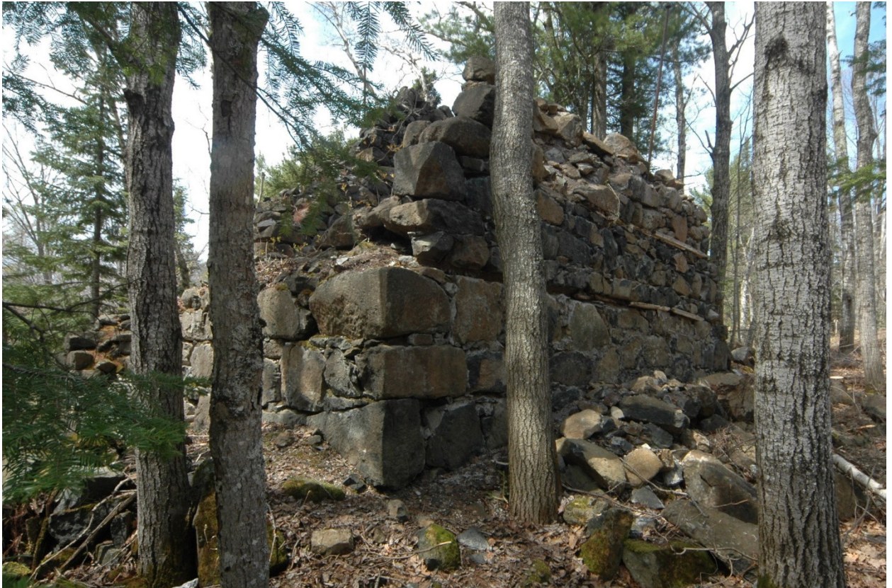
Figure 3.10. The Pennsylvania Mine Hoist House. (Image by author)
