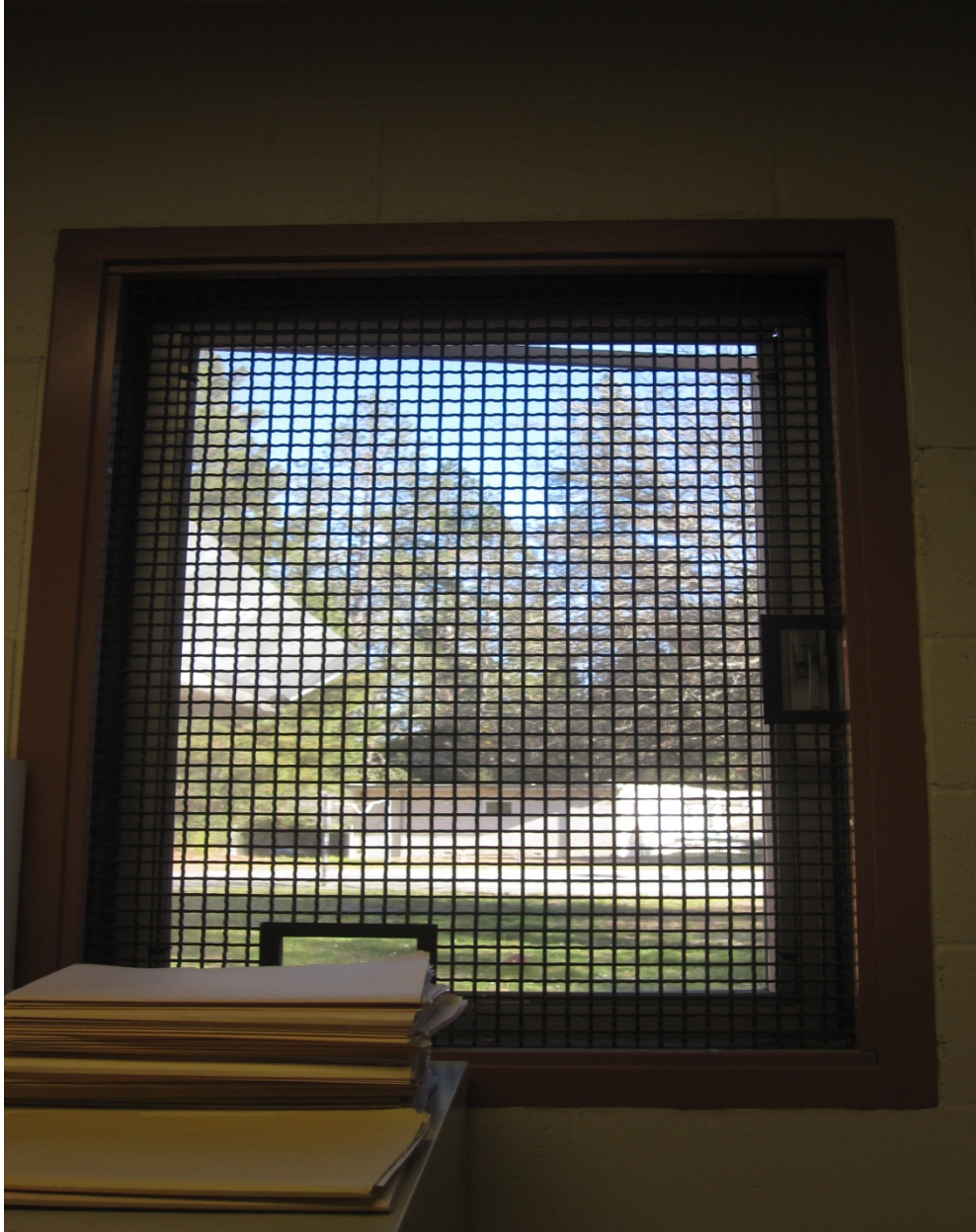
Photo 5. The windows of the classrooms are caged
