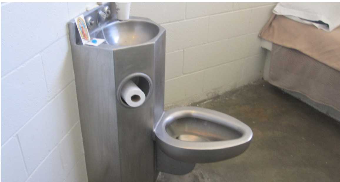
Photo 2. The small metal toilet/sink combination is inside the room.
