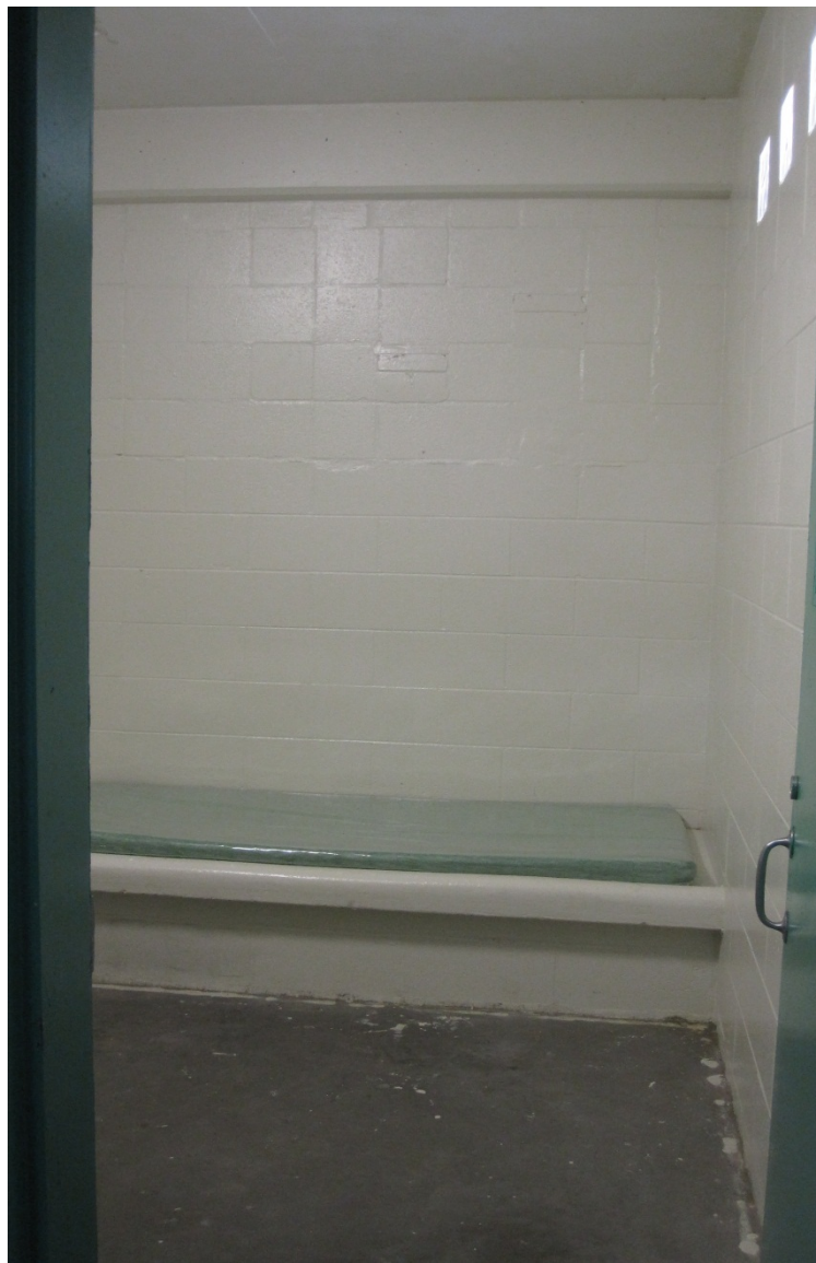
Photo 6. Isolation Room or “Solitary” room attached to A unit classroom
