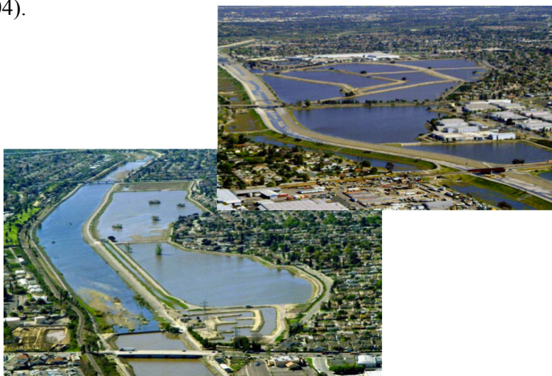
Figure 9: Rio Hondo (top) and San Gabriel (bottom) Spreading Grounds (Johnson, 2009a)
