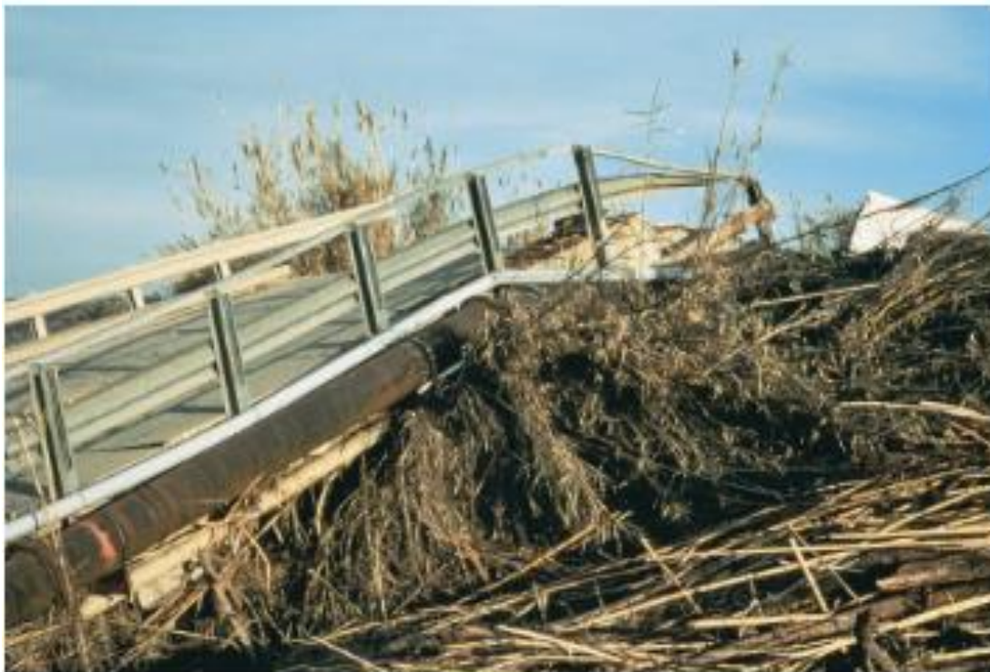
Figure 6. Dislodged A. donax stacked behind the River Road Bridge on the Santa Ana River from a 2004 flood (taken from Cal-IPC, 2011)
