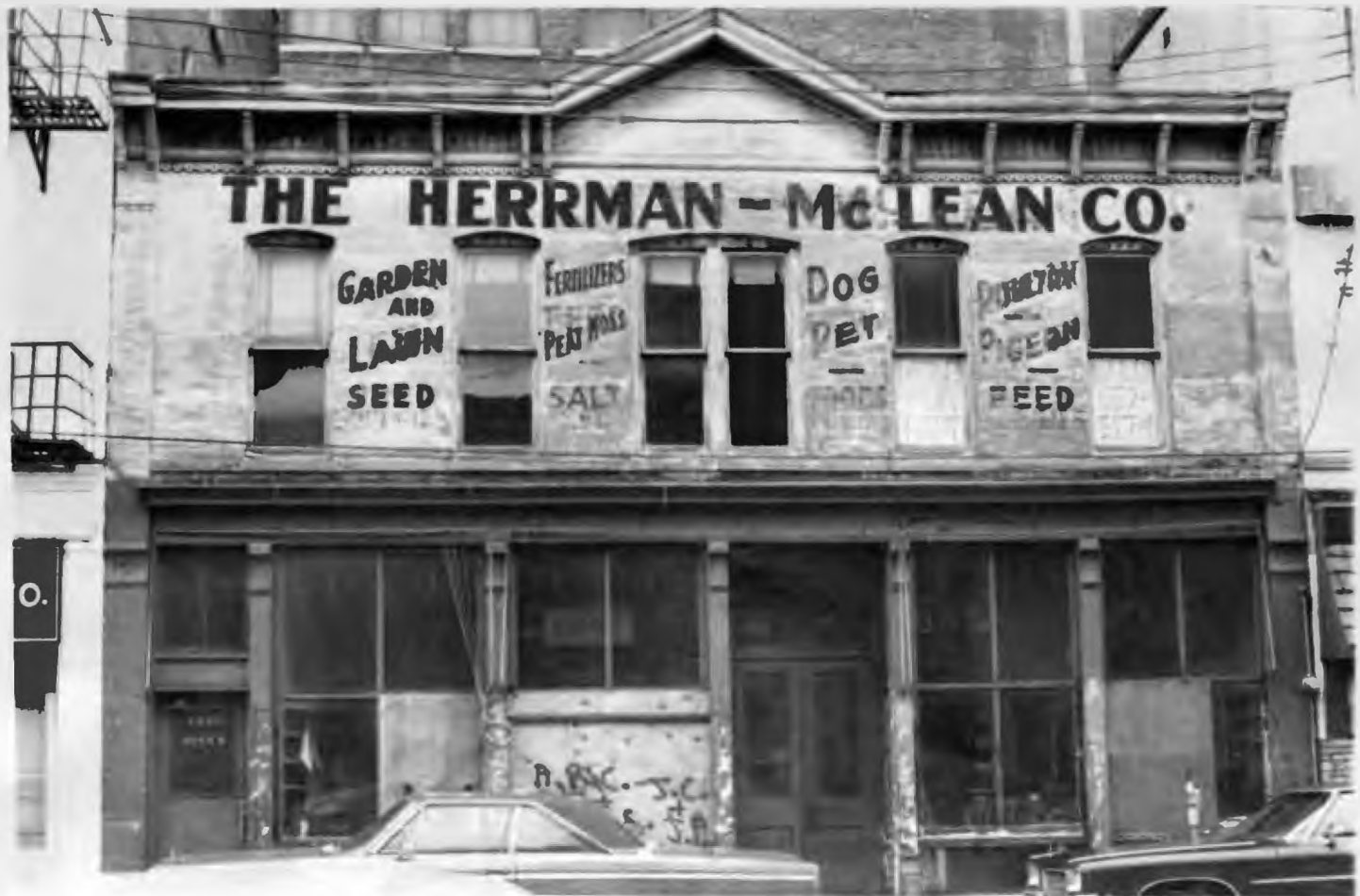
16. This fine commercial building, with its interior still intact, is currently unoccupied.
