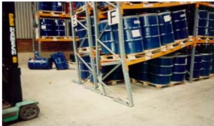
Figure 3.3: Failure of racking systems due to load and deformation built up [29].
