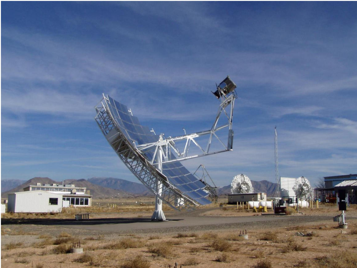
Figure 1. McDonnell Douglas dish, showing typical balanced configuration.
