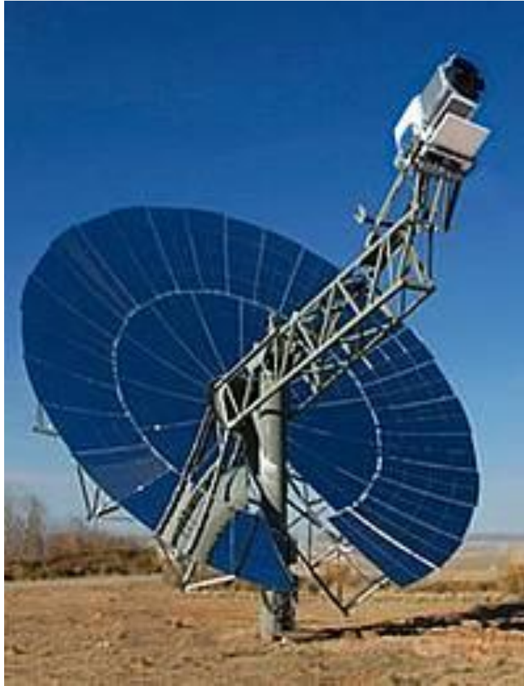
Figure 28. Balanced dish design with keyhole to accommodate pedestal.
