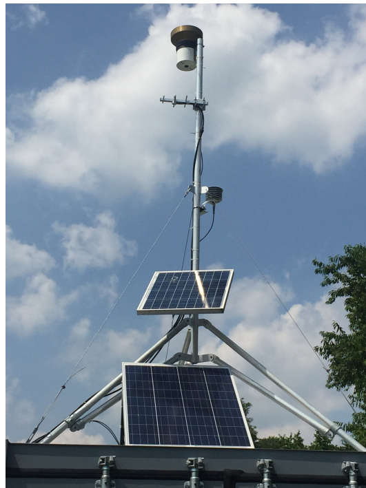
Figure 7. Weather station with 3 dB Yagi antenna for data transmission from the site.
