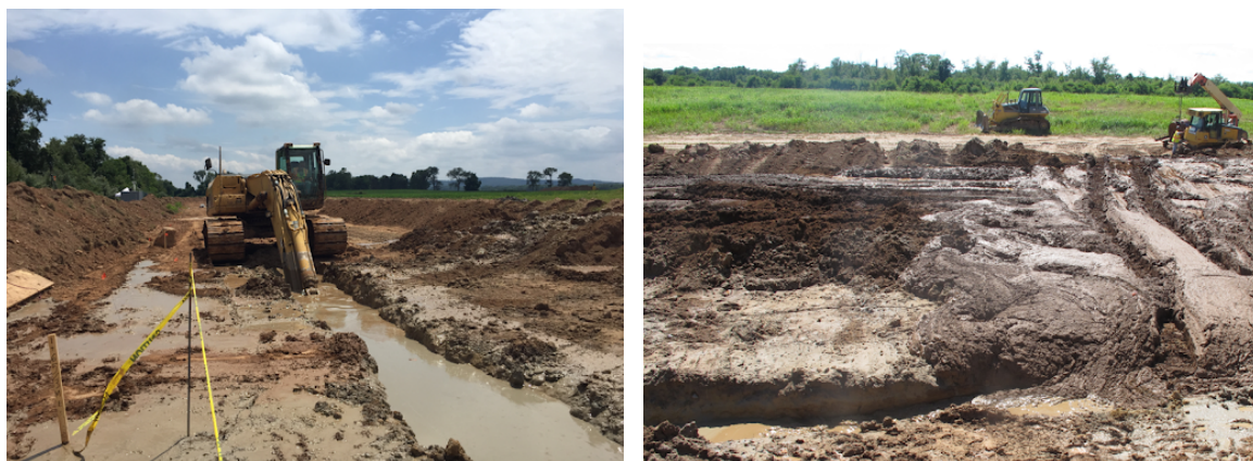
Figure 2. Excavation and Backfill at the test site.
