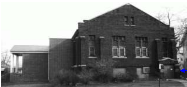
3248 DeSota Cleveland Heights. Photo taken 2001 shows addition completed in 2000 by current owner Congregation Beth El. Photo taken May 2006 By Jeffrey Morris
