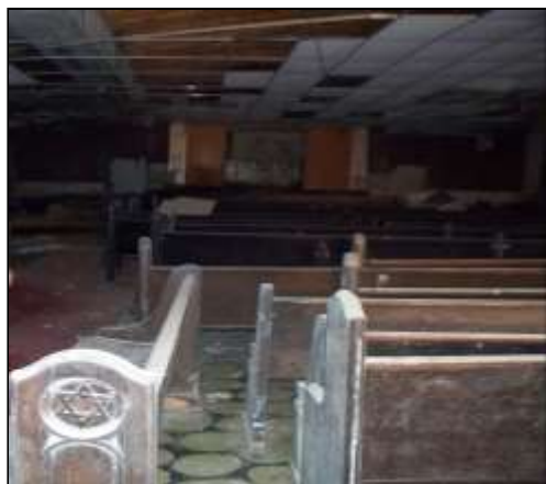
877 Parkwood Drive. Photo taken September 2011 showing years of neglect to the once beautiful Synagogue and Church. The drop ceiling shown was added after rafters were added that span the balcony. Those two ceilings are below a second drop ceiling that spans the high ceiling consisting of sky lights that were installed when the building was built in 1924. Demolished November, 2013
