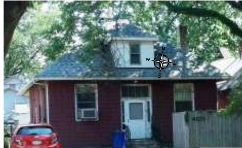
4101 John Street photo taken June 2012 Jeff Morris Note Plat map to the right shows, 4101 John as having a home towards the front of the lot, and a block building in the rear.
