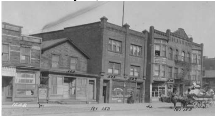
Photo of the 500 block of Hill St., taken April 1924 in preparation for the construction of train tracks into the rail station beneath the Terminal Tower. Source: Cleveland State University. Michael Schwartz Library. Special Collections
