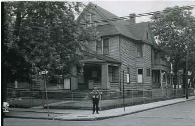
5702 Scovill Road. Purchased by Agudath B'nai Israel Anshe Sfard Romania in 1925. Sold in 1928. Source: The photo is part of a survey completed by the County Recorder in June 1959 of all non-commercial properties. The numbers held up by the sign holder are the Permanent Parcel Number.
