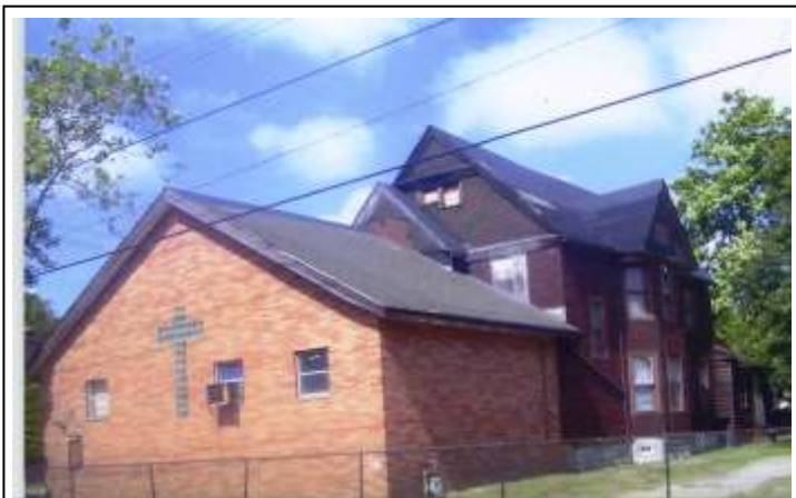
997 Lakeview Drive. Photo taken by Jeff Morris, May 2009. Former location of Ahavath Zion aka The Independent Ahavath Zion. The date the front of the building was added is unknown.
