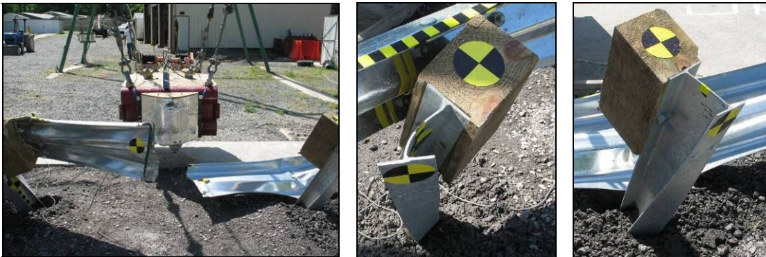
Fig. 11. Test 03-5: Overall damage (left) and post damage at splice (center) and non-splice location (right)
