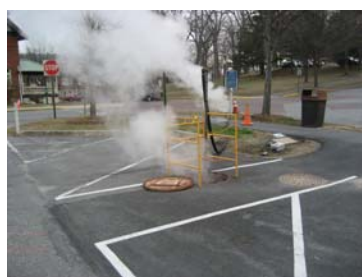
Figure 36: Hot storm water being removed from a manhole and pumped into a storm drain that flows directly into Miller Run (10 March 2008).
