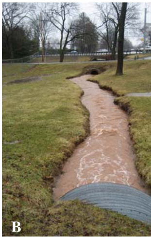
A, B: Downstream (A) and upstream (B) reach of the stream impacted by high sediment loads during 7-8 Mar 2008 rain event.
