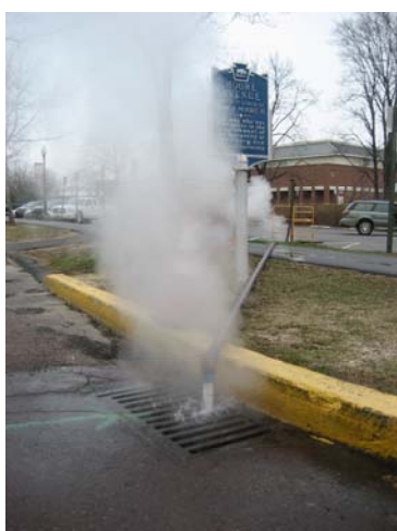
Figure 36: Hot storm water being removed from a manhole and pumped into a storm drain that flows directly into Miller Run (10 March 2008).
