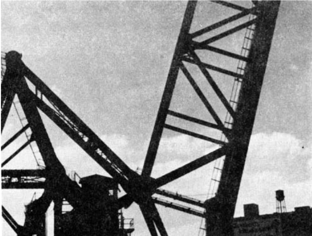
XVII. Detailed in silhouette of the present Columbus Road Bridge in the open position.
