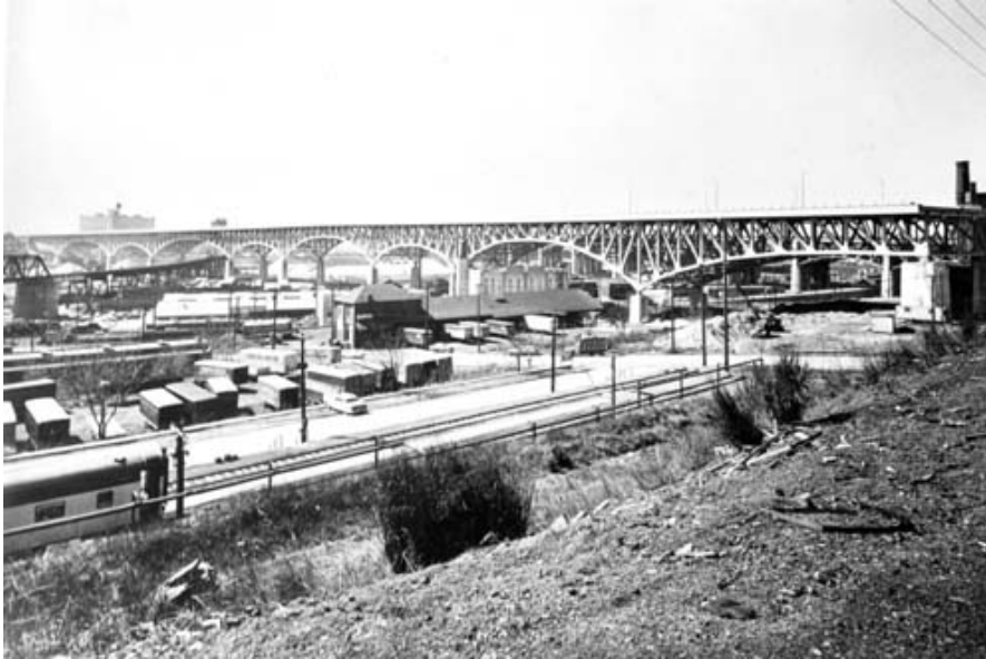
Figure XI. The Inner Belt Bridge, the widest bridge ever built in Ohio
