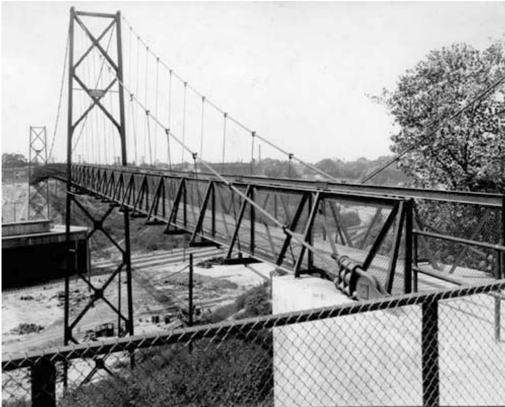
Figure XXIX. The Sidaway Bridge over Kingsbury Run is Cleveland's only suspension bridge.
