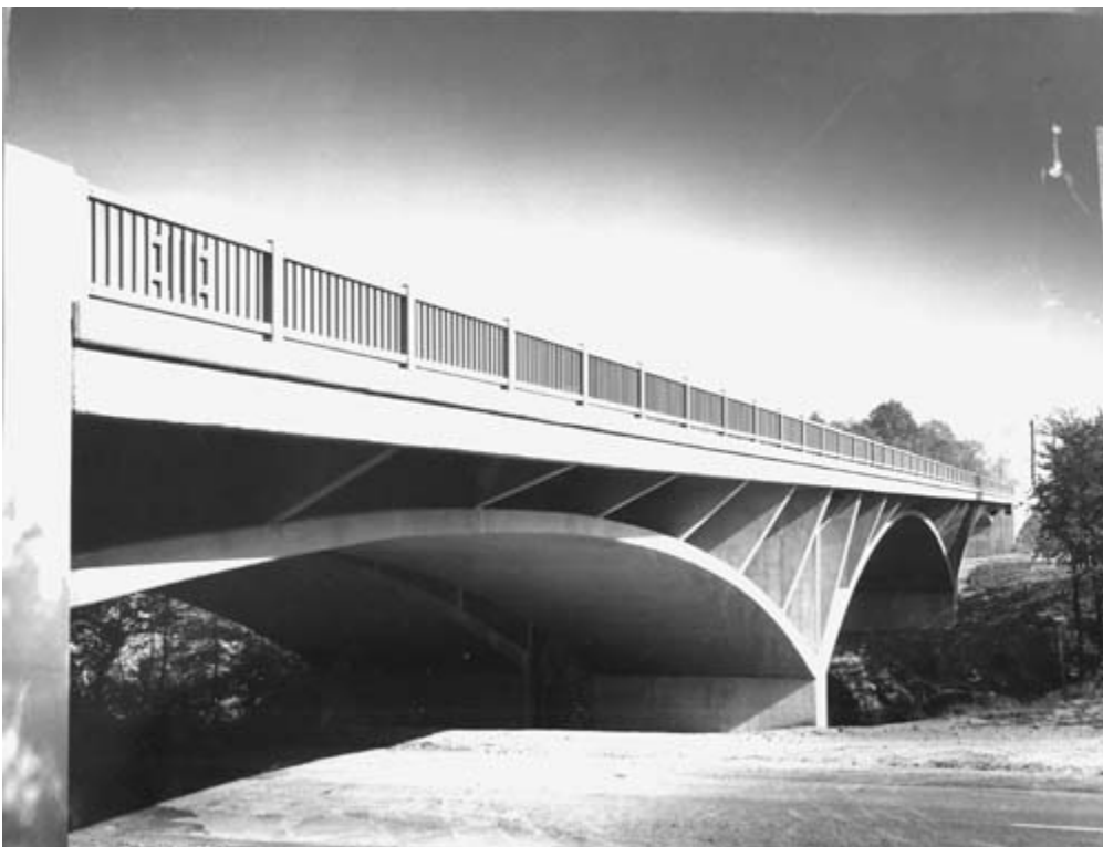
Figure XX. The graceful concrete arches of the Monticello Bridge.
