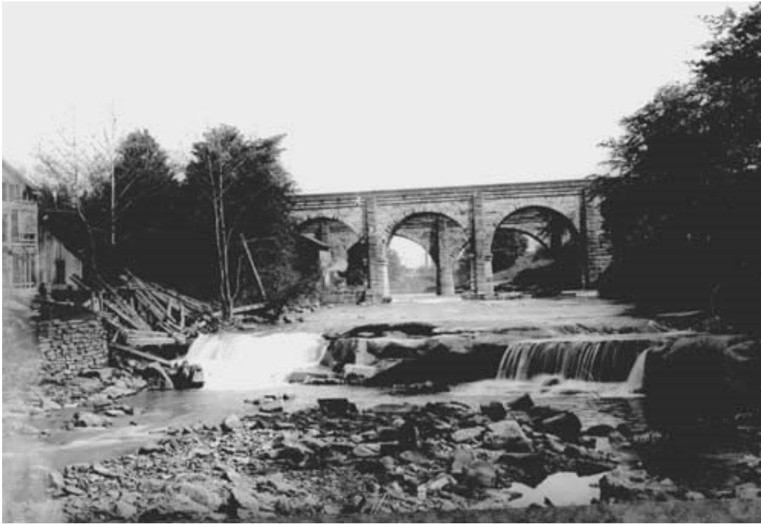
Figure I. Original Lake Shore & Michigan Southern Railroad and Cleveland, Columbus, Cincinnati Railroad Bridges built about 1850 and still standing near Berea, Ohio.
