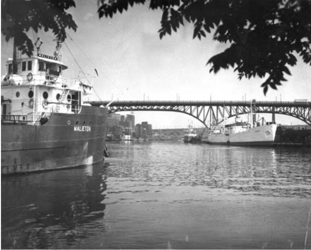
Figure XXXI. Main Avenue Bridge today, looking south toward the Detroit-Superior Viaduct.
