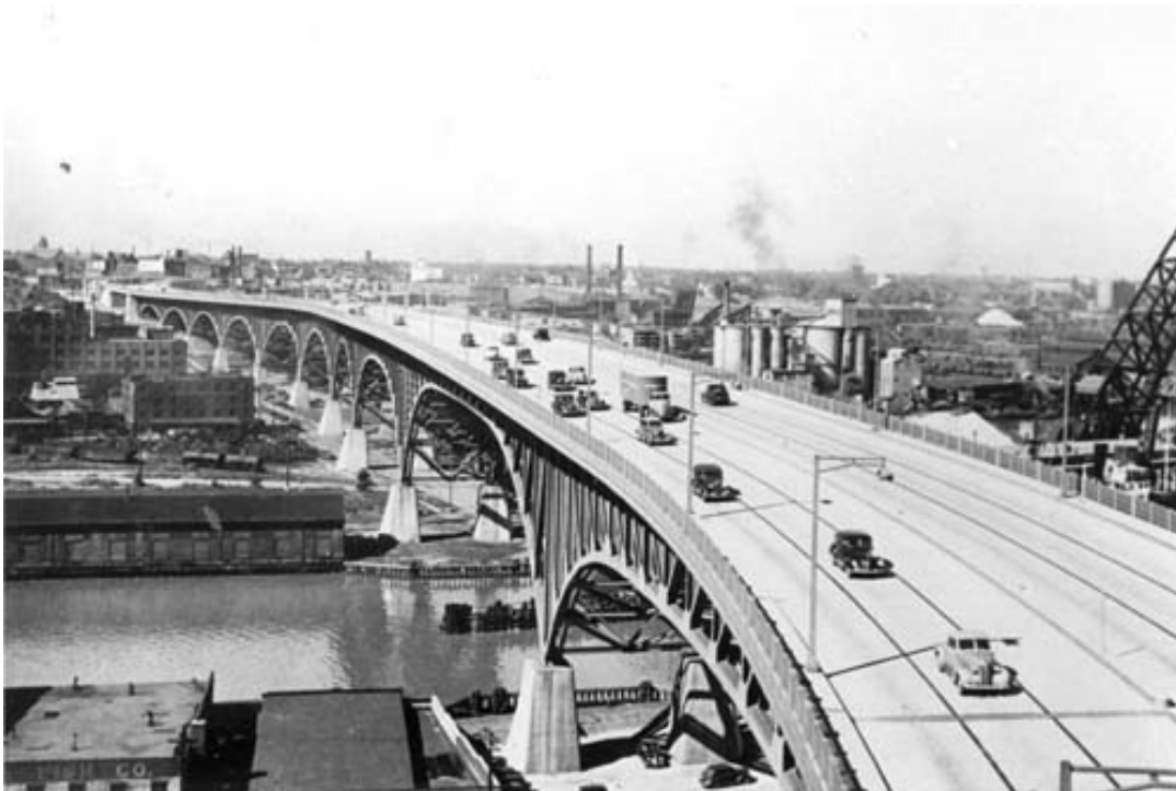
Figure II. The Main Avenue Bridge shortly after its opening in 1939 with the first installation of Sodium Vapor lighting in the United States.
