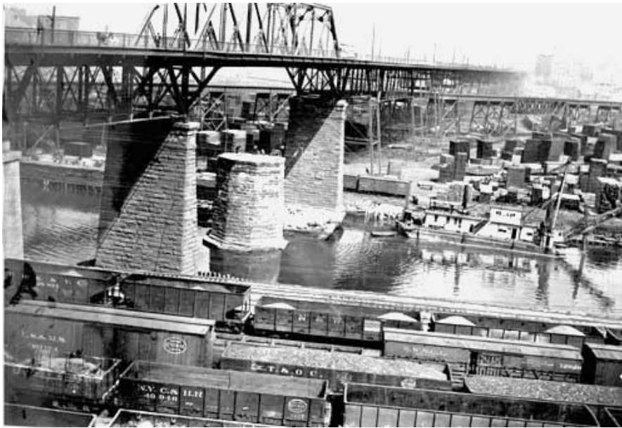
Figure X. Central Viaduct showing the fixed span that replaced the old movable span.
