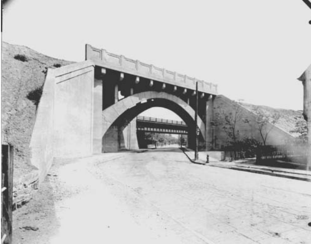
Figure XXVIII. A concrete arch railroad bridge over East 92nd Street is now a part of the Cleveland area RTA system.
