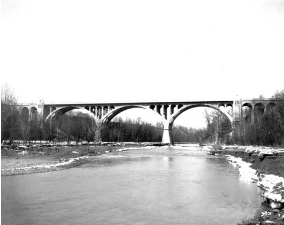
Figure XXV. The Hilliard Road Bridge over the Rocky River, built in 1926 with A.M. Felgate the engineer.
