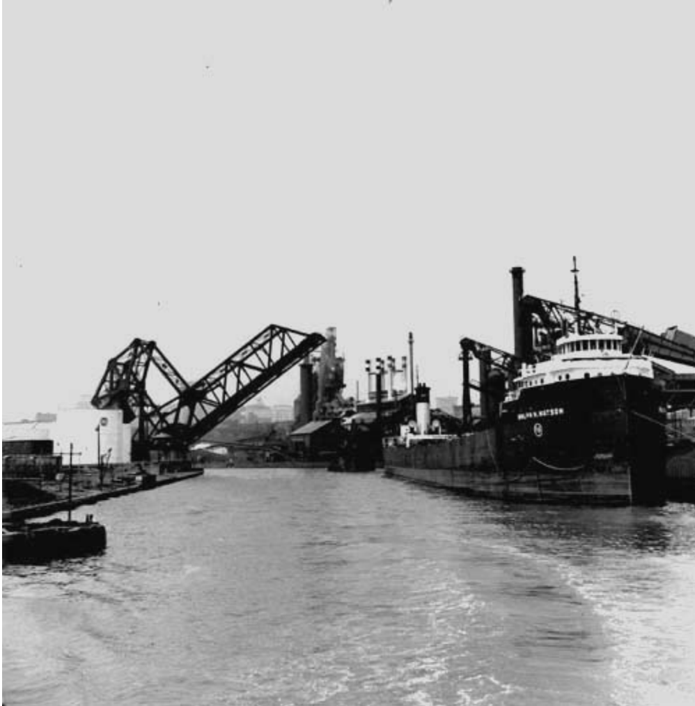
Figure XXVII. A jackknife bridge in the open position to allow passage of an ore boat on the Cuyahoga River.
