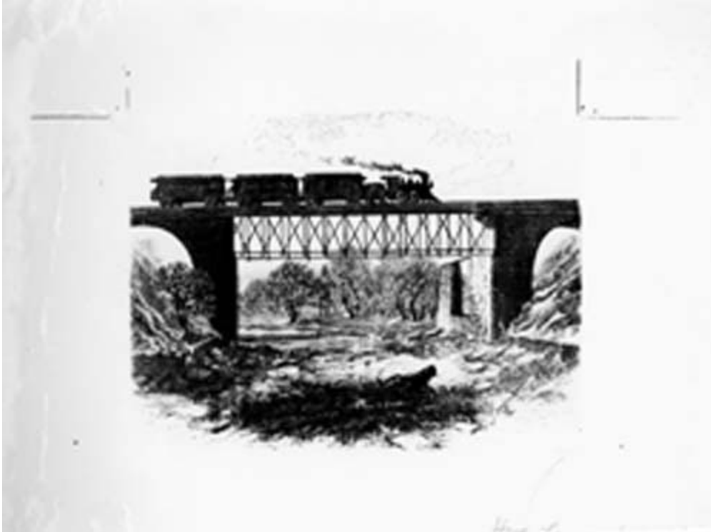
Figure XVIII. Ashtabula Bridge on the Lake Shore and Michigan Railroad, scene of one of the worst railroad disasters in U.S. history.
