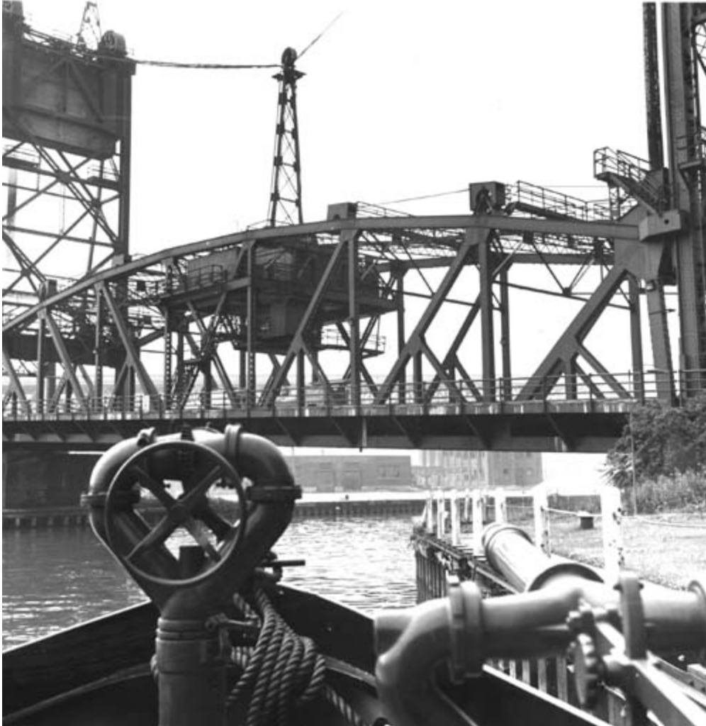
Figure XIII. Vertical Lift Bridge in operation at Eagle Street
