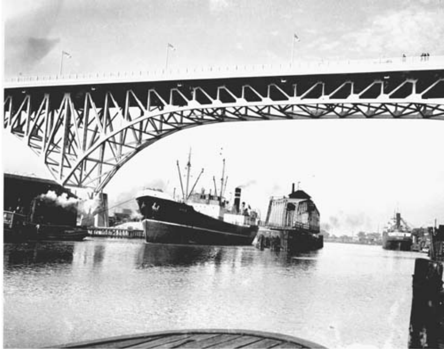
Figure IX. Main Avenue Bridge with the old Main Avenue Swing Bridge in the open position.
