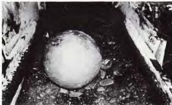
One of the extremely hard concretions encountered in the Milo-Grogan Outfall Area Storm Relief Sewer project in Columbus.
