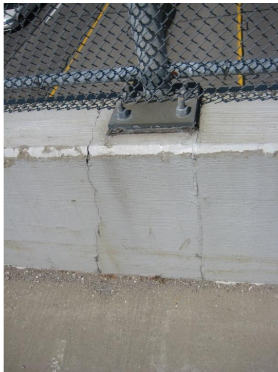
Figure 19: Completely sealed joint located directly below VPF base plate, Wagar Road
