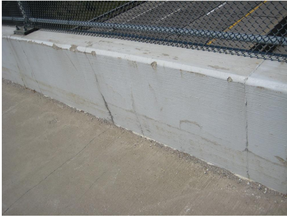
Figure 15: Crack below VPF base plate, Wagar Road
