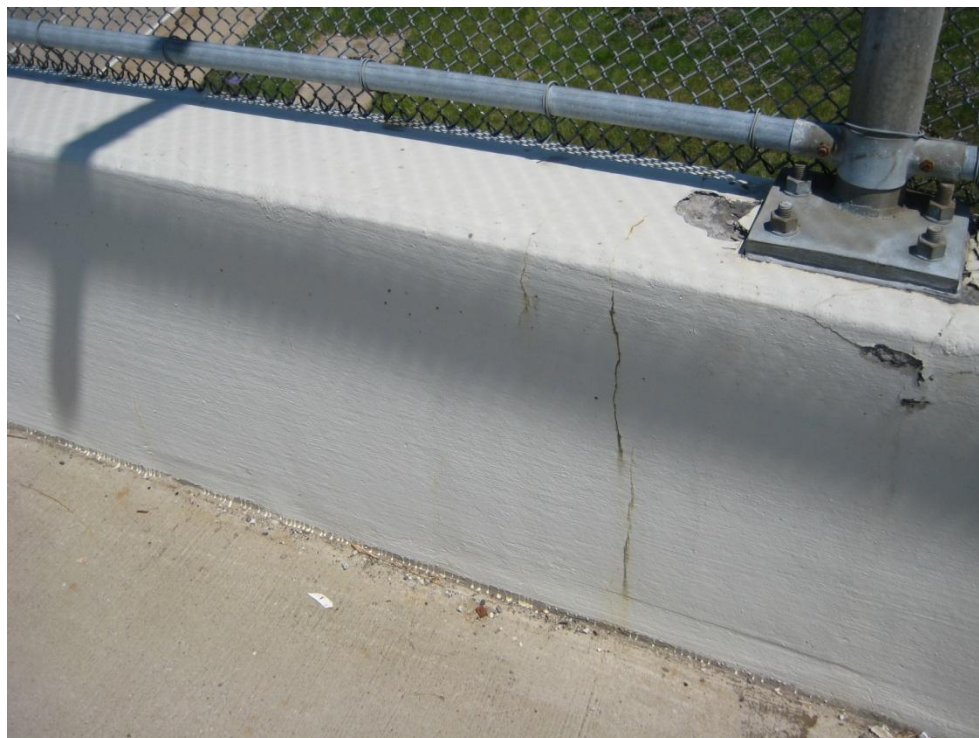
Figure 13: Cracking and flaking below VPF base plate, Spring Road
