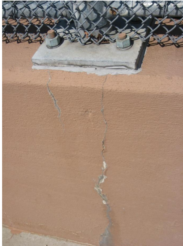
Figure 11: Crack below VPF base plate, Sheldon Road
