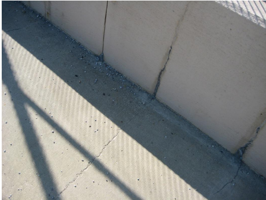
Figure 22: Continuous crack through sidewalk, Wagar Road
