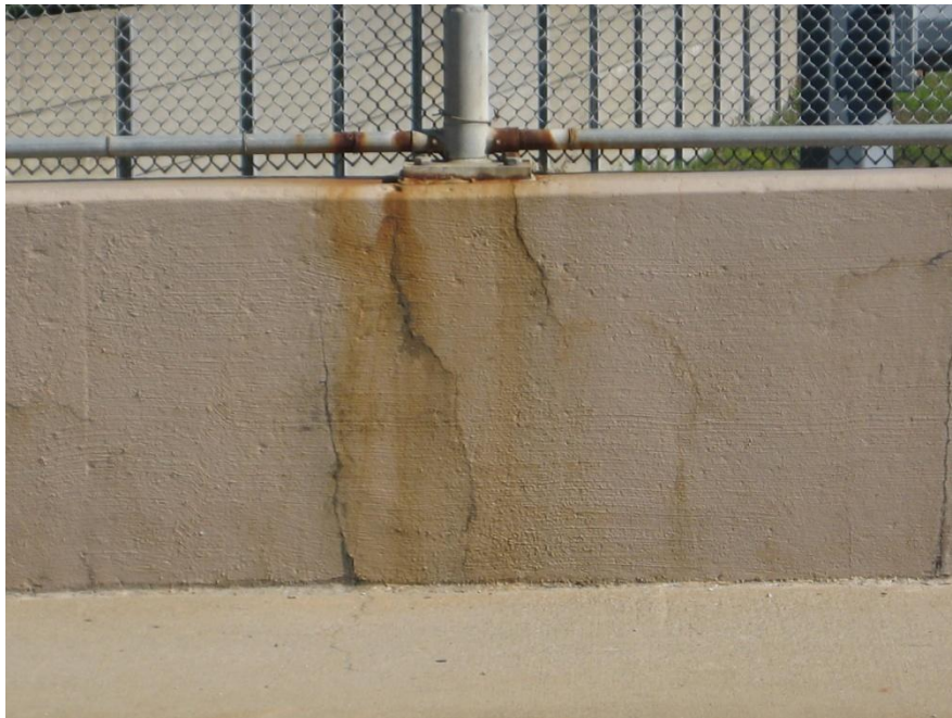
Figure 11: Crack below VPF base plate, Sheldon Road
