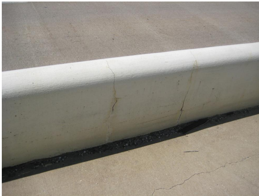
Figure 13: Cracking and flaking below VPF base plate, Spring Road
