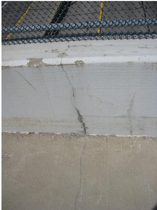
Figure 22: Continuous crack through sidewalk, Wagar Road
