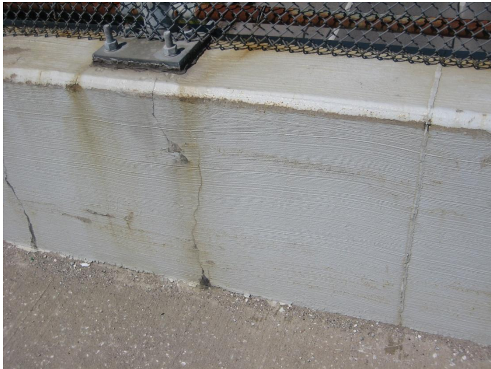
Figure 15: Crack below VPF base plate, Wagar Road
