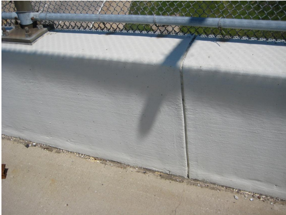
Figure 19: Completely sealed joint located directly below VPF base plate, Wagar Road
