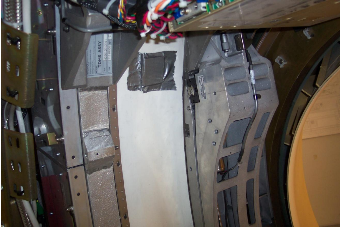
Figure 53: Copper Strips Taped to End of Detector System
