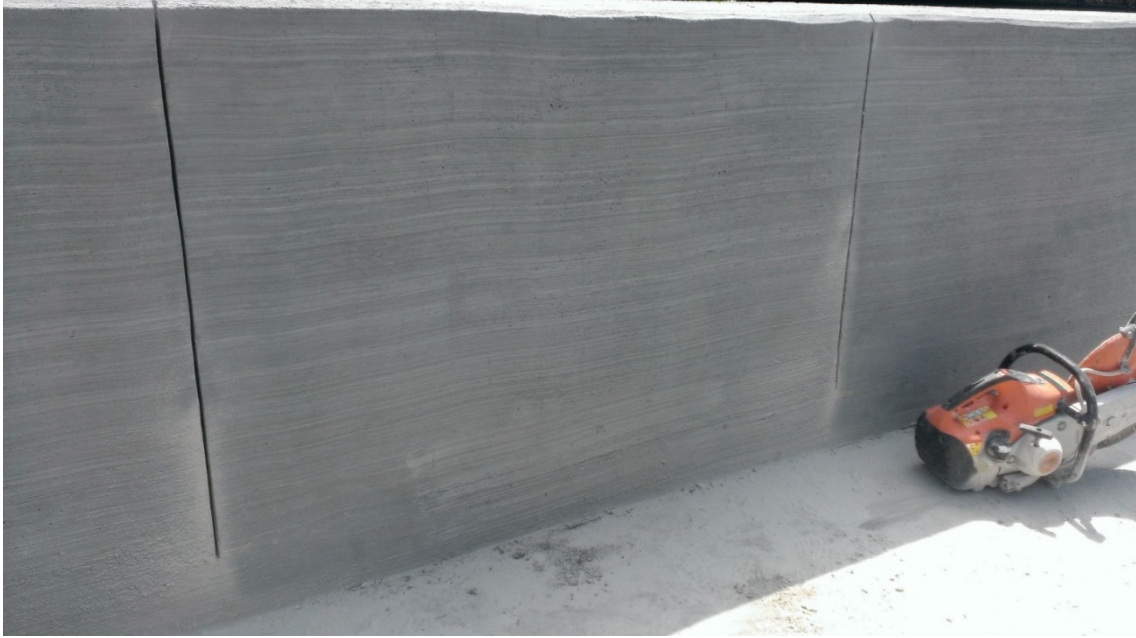
Figure 1: Finished Bridge Parapet (Photo Provided by Lauren Hedges)
