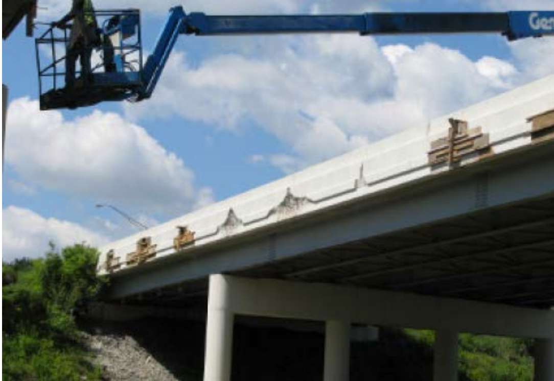
Figure 29: Bridge Number GRE-42-0789 (Photo Provided by Brandon Collett, PE)
