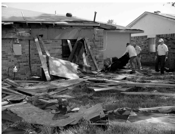
Figure 3. Roofing Debris: Barrier to Electricity Restoration. An elderly couple was denied electrical hookup until debris was cleared.
