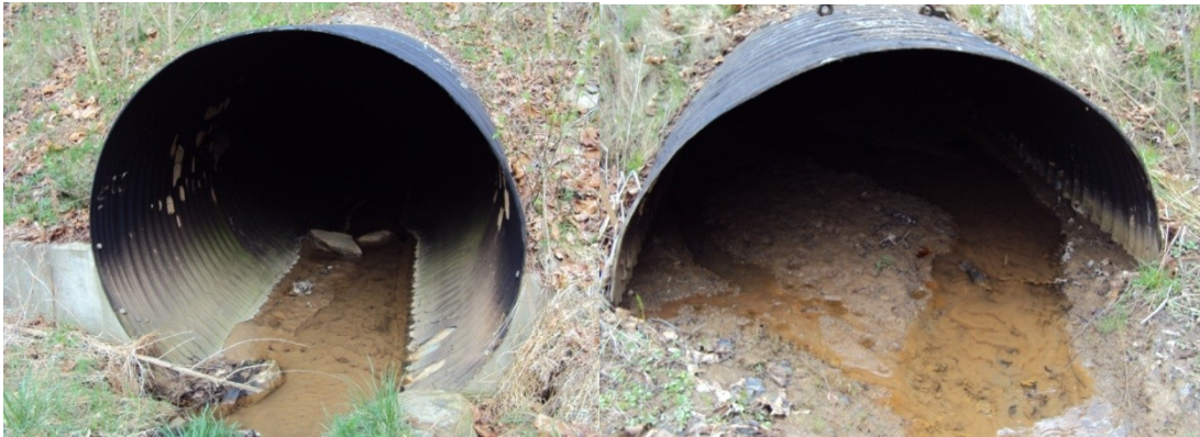
Culvert 5F Inlet
