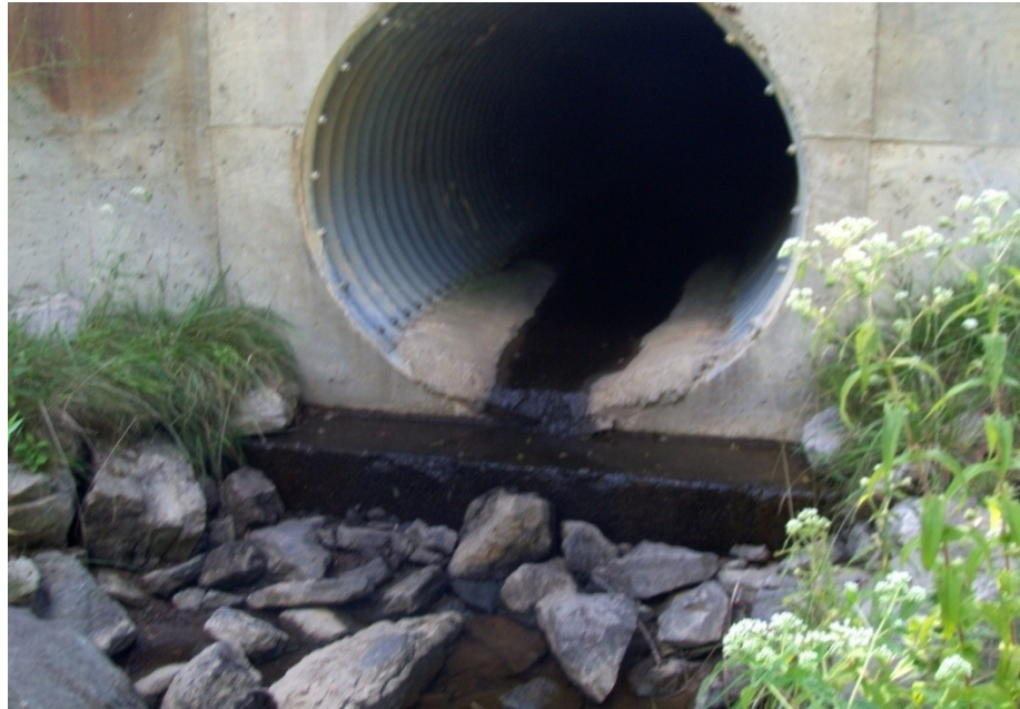
Figure 4.3 Culvert 2A, showing concrete lining on bottom of culvert
