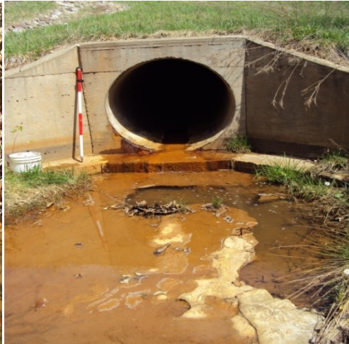
Water exiting culvert 2E
