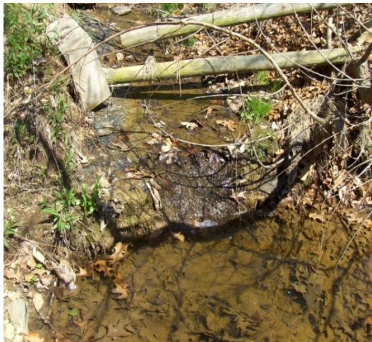
Water upstream of culvert 2E
