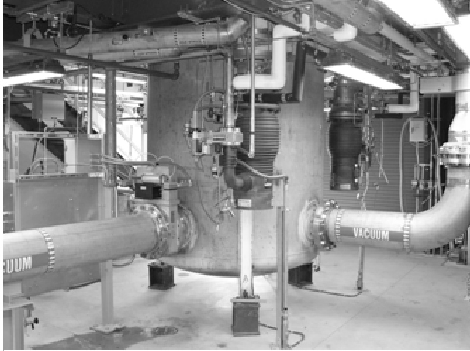
Figure 12 – Bottom view of SMIRF vacuum chamber
