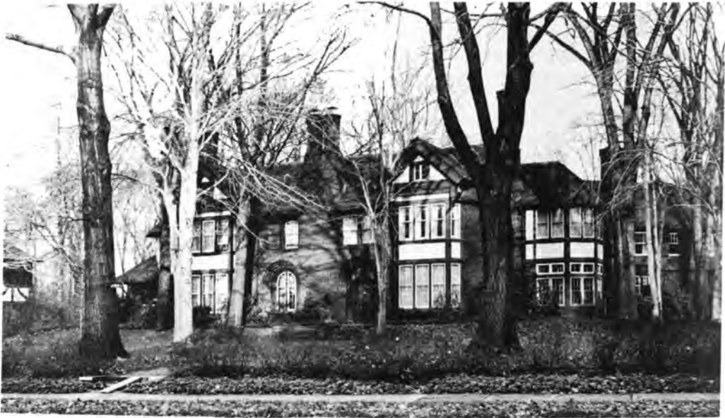
Fig. 1: Cashman House, Shaker Heights. The composition focuses its strictest discipline on the center of the facade; the ends are more freely balanced.
