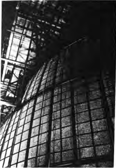
Plaster-and-steel "sky dome" (since removed) seen from backstage floor, made an effective theatrical backdrop but deadened sound.
