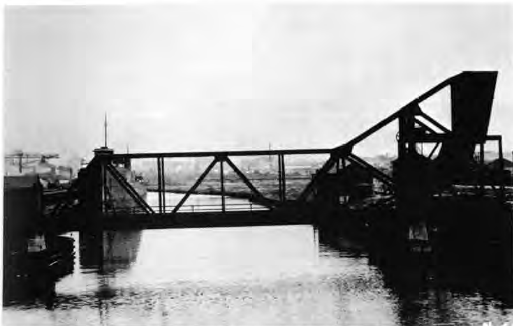
Scherzer Rolling Lift bridge over the Cuyahoga River, built for the B&O Railroad.
