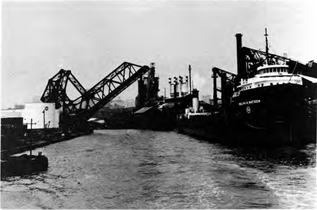
Jack-knife bridge allows freighter to pass up the Cuyahoga River (Bridge No. 19, Erie Railroad).
