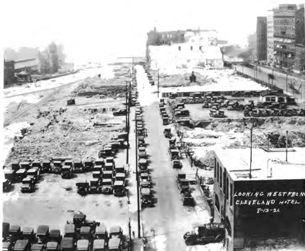
Looking west from Hotel Cleveland, August, 1926. The future site of part of the station after clearing but before excavation. Note streetcar slit in middle of Superior Avenue, leading to a lower level of the Detroit-Superior Bridge. CSU Archives.
