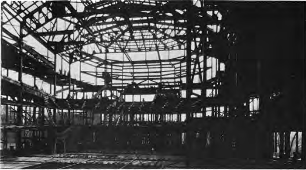
By March 10, 1930, structural steel encloses the main auditorium.
