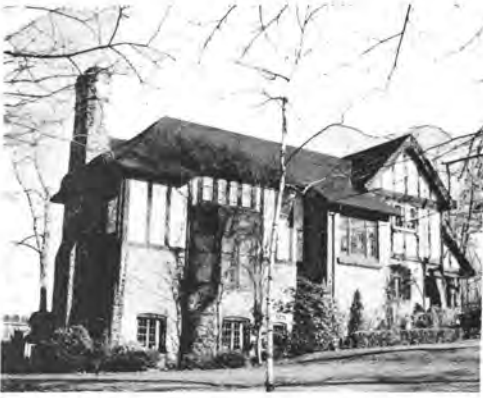
Fig. 12: Dan Hanna House parkway facade. The stonework is the chief decorative interest of this facade, the fine depressed arches of the windows, the magnificent chimney at the end of the house and the beautifully precise angle buttresses, split by the angles of the house.
