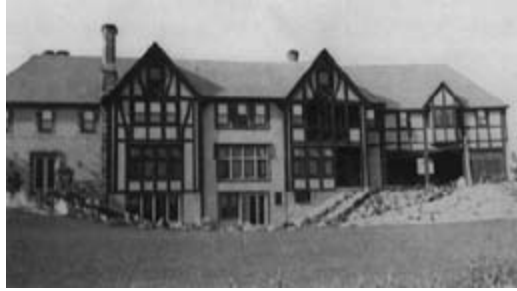
Bourne Home under construction at 2800 Selkirk Road. Photo taken early 1920's. Courtesy Mr. Cal Bourne.
