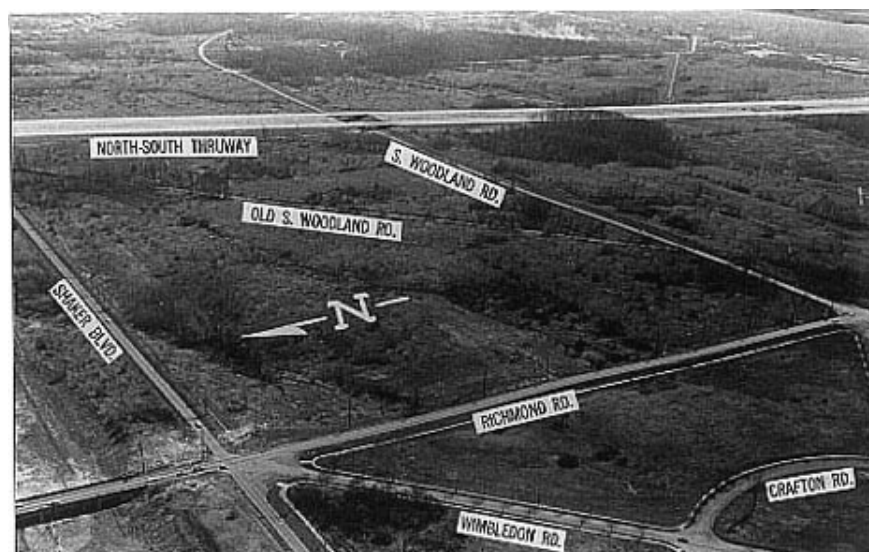
1962 Site of proposed Shopping center on Richmond Rd. and South Woodland Courtesy of the Cleveland Press Collection held at Cleveland State University
