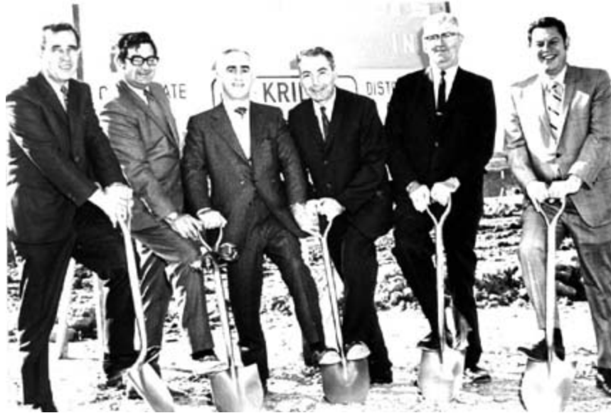
Groundbreaking for Fabri-Centers' new distribution center at 23550 Commerce Park Road. September 1969. Left to Right Leonard Krill, Contractor, Keeva Kekst, Architect, Martin Rosskamm, Fabric Center President, Mario Frato, Building Inspector, John Havel, Police Chief, Harvey Friedman, President of Council.
