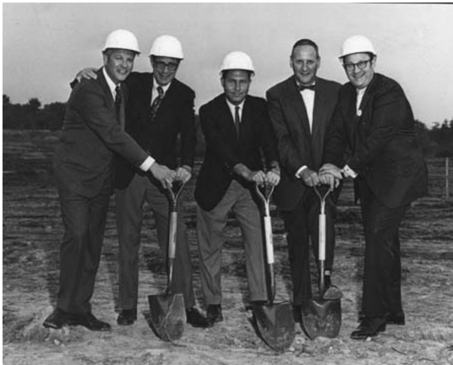
The groundbreaking for The Temple Branch" Left to Right. Lionel Greenbaum co-chair of the fundraising committee, Charles Evens, Chair of the Building committee, Robert Deutch, co-chair of the fundraising committee, Bud (Max) Eisner, president of the Temple, Ernest Siegler member and contractor.
