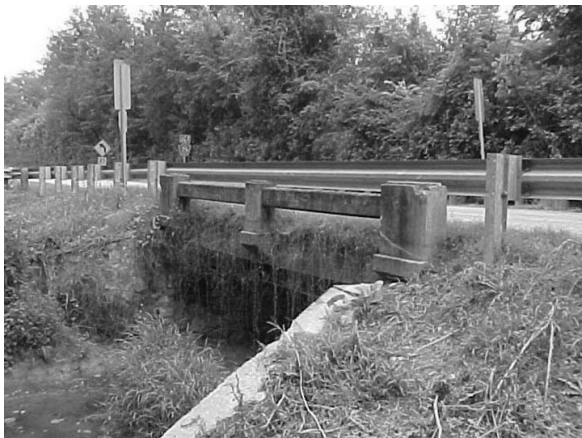
Fig. 3: Shelby county bridge no. 020-59-202Z
