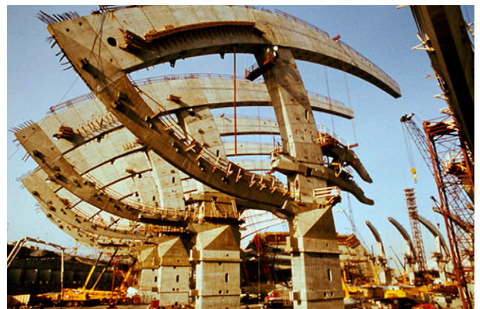
Fig. 6. Ribs of the Olympic Stadium (Parc Olympique Quebec 2011; credit: Olympic Park of Montréal)
