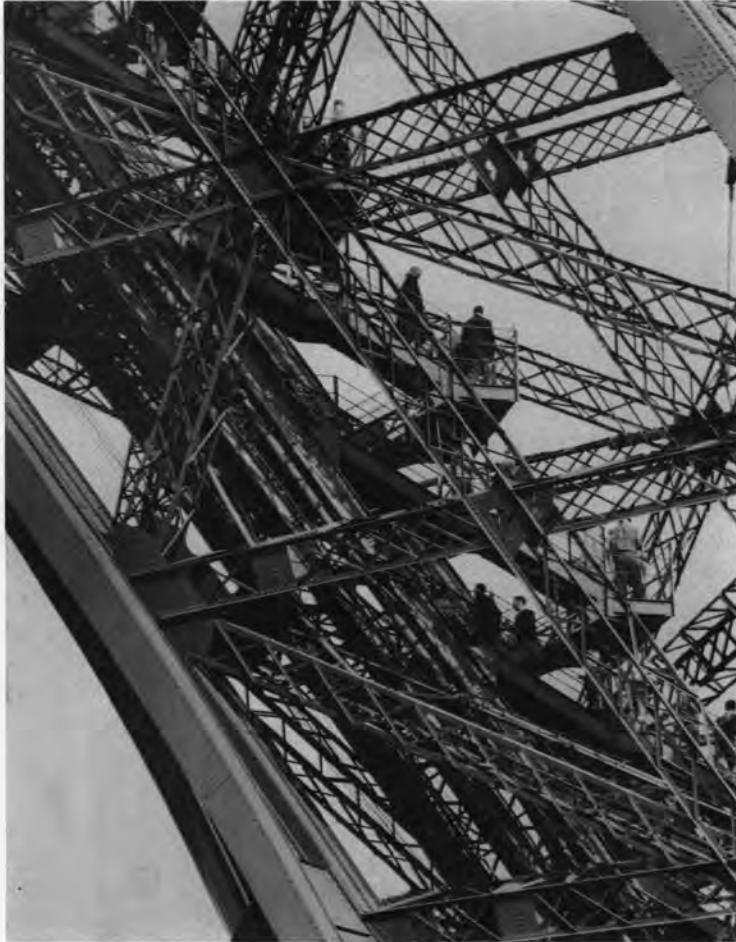
Stairway up the tower. Photo courtesy of The Cleveland Press Collection, Cleveland State University Archives.
