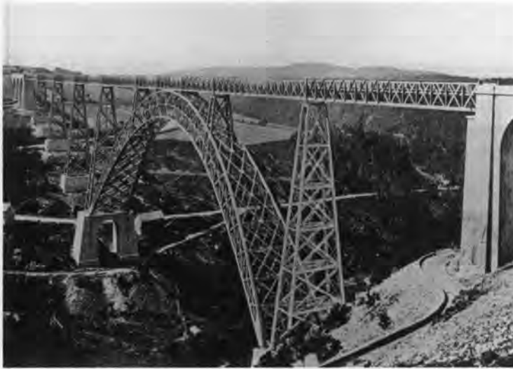
Eiffel first won fame as a builder of bridges. At left: his monumental viaduct over the Truyère River at Garabit in the Massif Central of France—400 feet high, the highest in the world when it was built.
