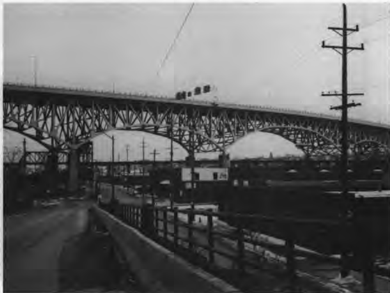
Upper photo: steel bridges give a light, graceful appearance to elevated portions of the 8-lane Innerbelt, such as this one over rail tracks and the Cuyahoga River. Lower photo: driving through the I-77/I-480 interchange is a stimulating three-dimensional experience.
