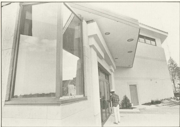
The recreation center is now in its final stages of construction.
