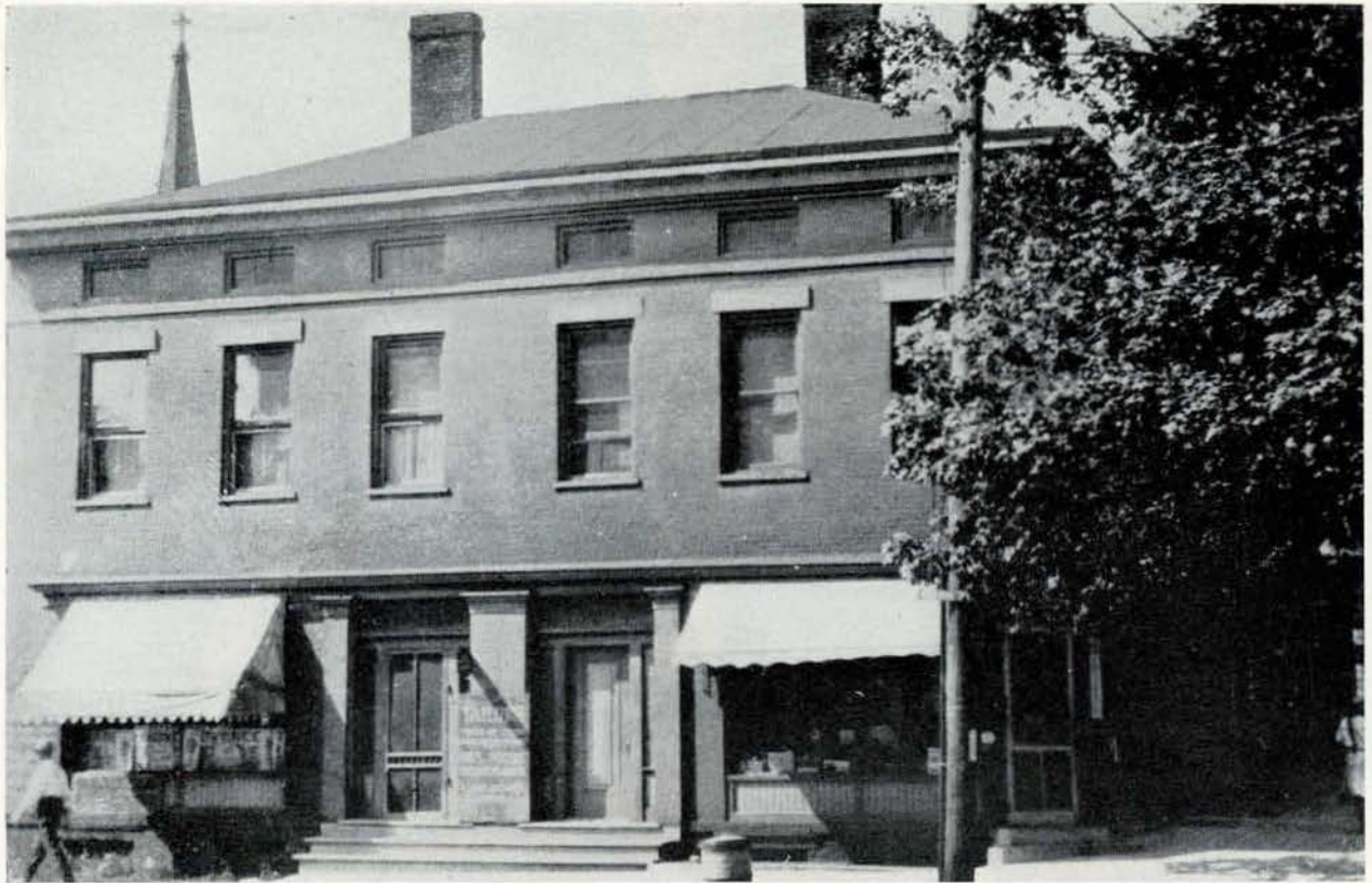
The double house on Oneida Street, occupied from 1850 to 1852. Classrooms were in the basement and on the first floor, laboratory and library on the second floor of the left half of the building. The right half housed the Boarding Department. The house then stood considerably higher above grade.
