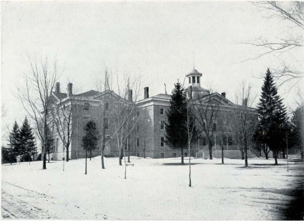
DOWNER COLLEGE AFTER REMODELING
