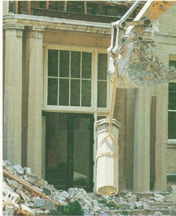
Deconstructing Stephenson Hall
