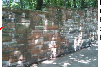
Mayfield Rd retaining wall. Built 1928 of LVC- quarried Euclid Bluestone.
