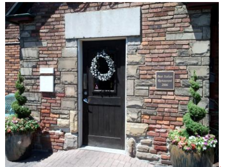
Montenerodomo clubhouse, 2198 Murray Hill Rd. Built 1937 with Euclid Bluestone accents. Now Michelangelo's restaurant.
