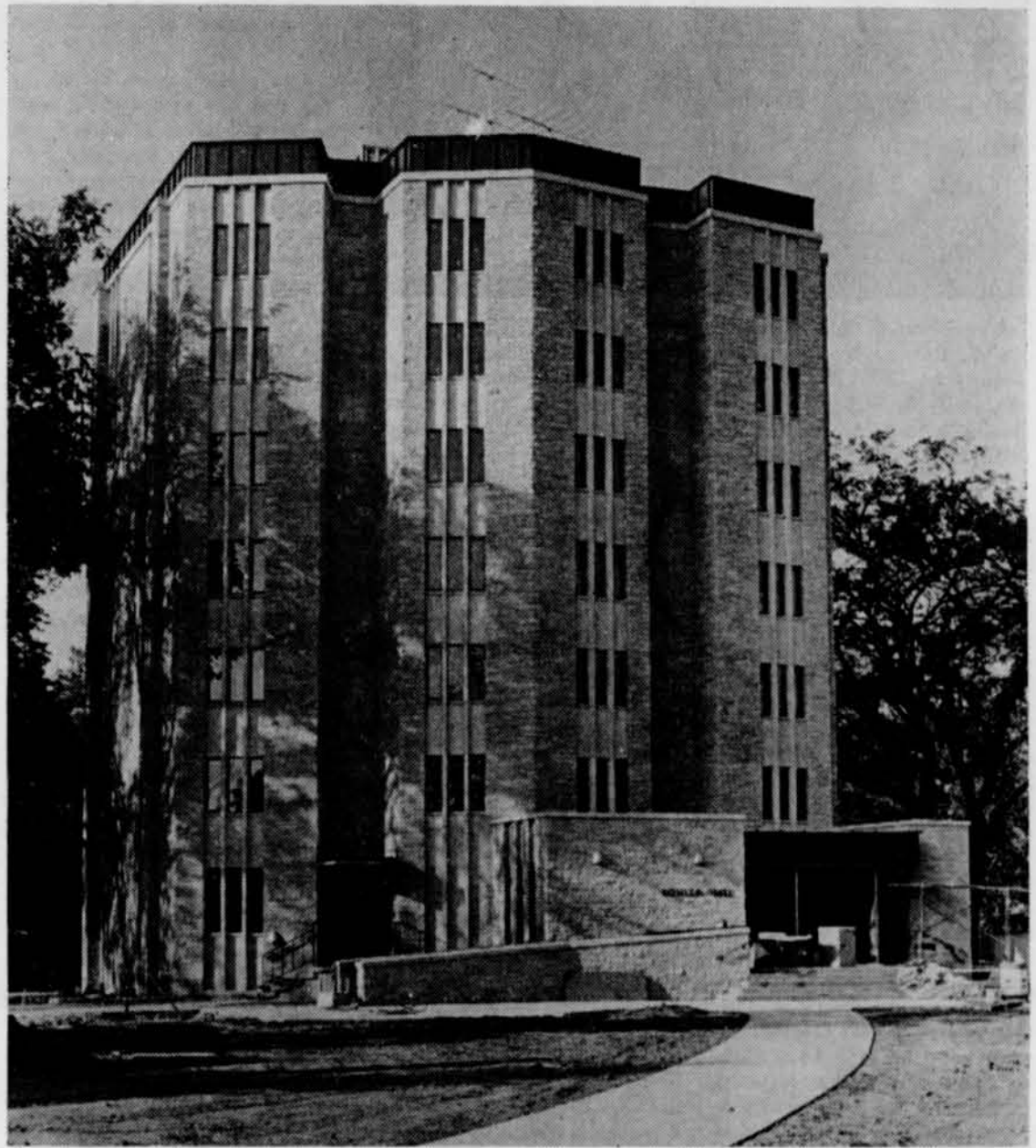
A NUMBER of skeptical senior women were delighted this week to find that the Ruth de Young Kohler Hall for women had been complete on schedule. The excellent summer weather here and the diligence of the prime contractors, Oscar J. Boldt Construction Co., Inc., both contributed to the speedy completion of the seven-story structure.
