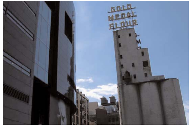
A view of the exterior of the new Guthrie building (left; G.B. Shaw's forehead is visible), overlooking one of the historic flour mills in the area near the theatre.
