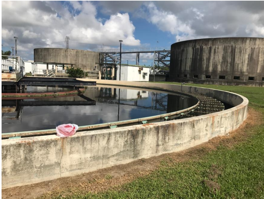
Figure 22. Secondary clarifier at Bridge City WWTP.
