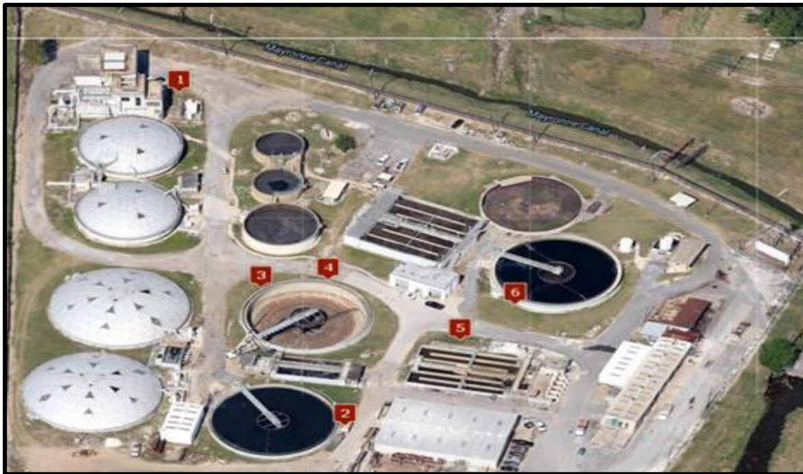
Figure 12: Marrero WWTP with monitoring locations
