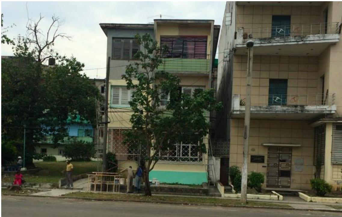
Figure 3 Paint crews at work on Avenida 20 de Mayo (Griffith, 2016)
