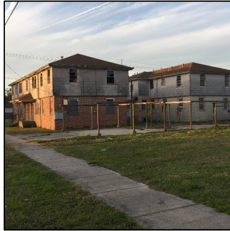
Figure 14. Abandoned 4-plexes across from the Macaluso home.
