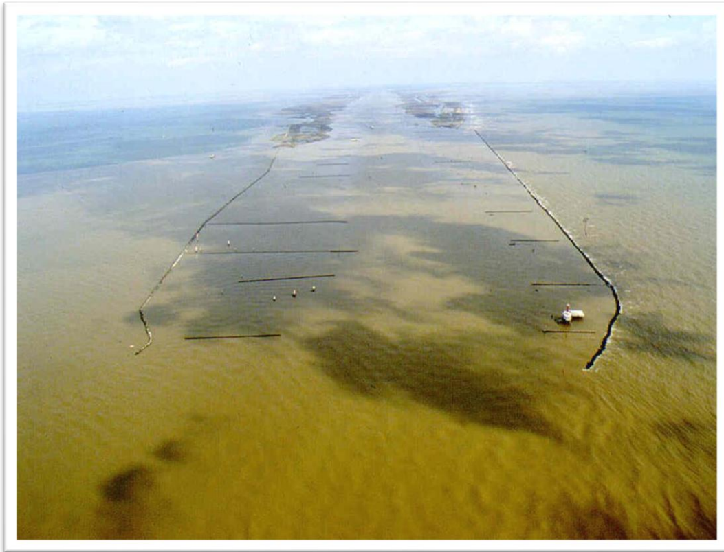
Figure 1-5 Southwest Pass Entrance showing rock jetties and timber pile dikes, date unknown (source: U. S. Army Corps of Engineers, New Orleans District)
