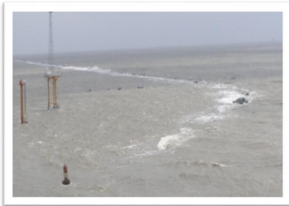
Figure 1-5 Southwest Pass Entrance showing rock jetties and timber pile dikes, date unknown (source: U. S. Army Corps of Engineers, New Orleans District)
