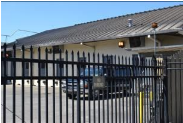
Fig. 3: Loading Dock, 04/03/2014, Elizabeth Major
