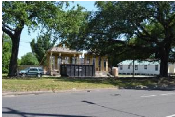
Fig. 6: Hurricane Damage on Bolivar, 04/03/2014, Elizabeth Major
