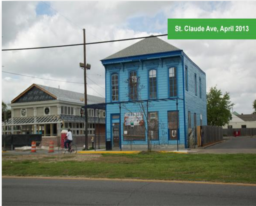
Figure 12: Renovations Occurring on St. Claude Avenue & St. Roch, 2013
