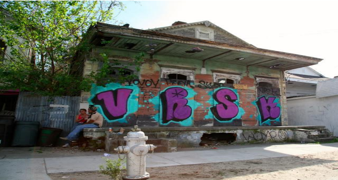
Figure 4: "Saint Claude Avenue Abandoned Residence, 2013
