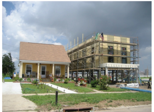
Figure 5 : The Make It Right project’s pink houses. Source: Thomas (2006).
