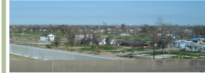
Figure 2: The Lower Ninth Ward & the improved levee. Source: Thomas (2007).
