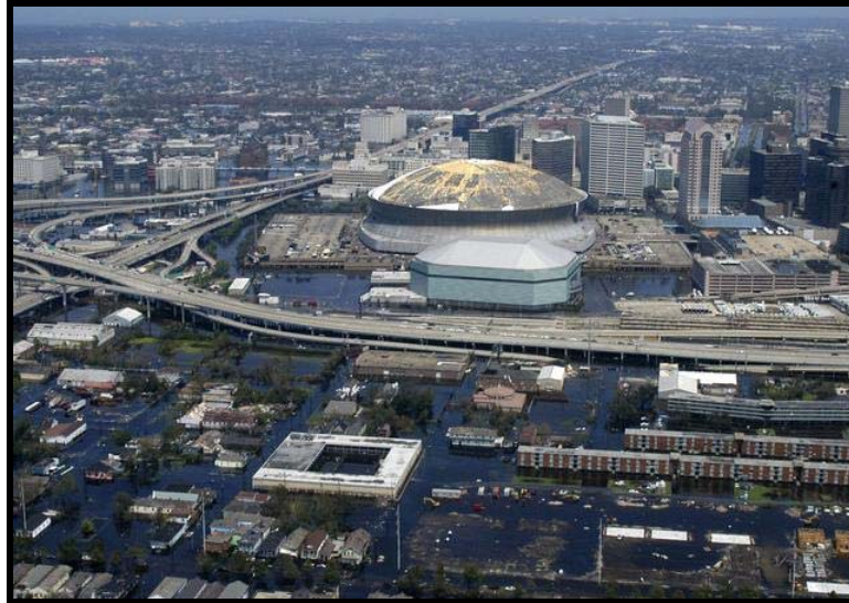
Figure 4 Extent of Katrina flooding (see online version for colours)
