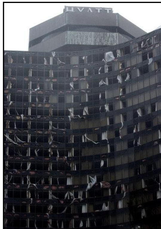
Windows blown out Hyatt Regency Hotel after Hurricane Katrina
