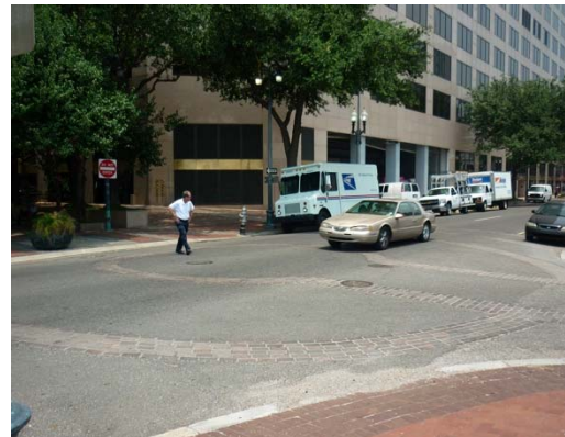
Figure 38: Brickwork along Lafayette Street.
