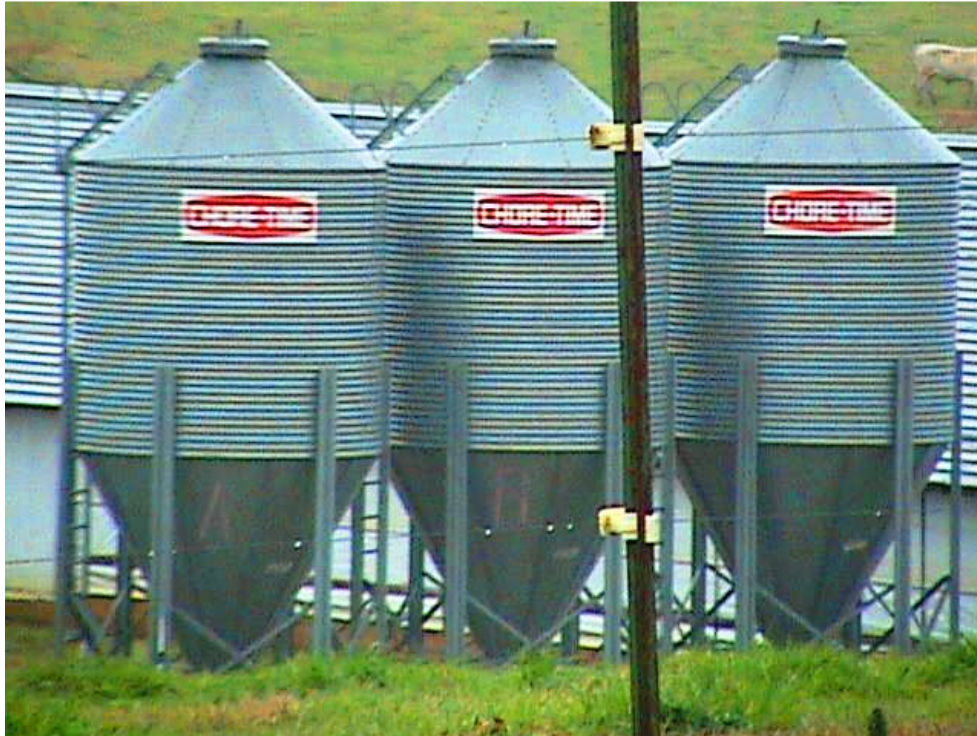
Illustration 3: Feed Silos at a CAFO in Mississippi
