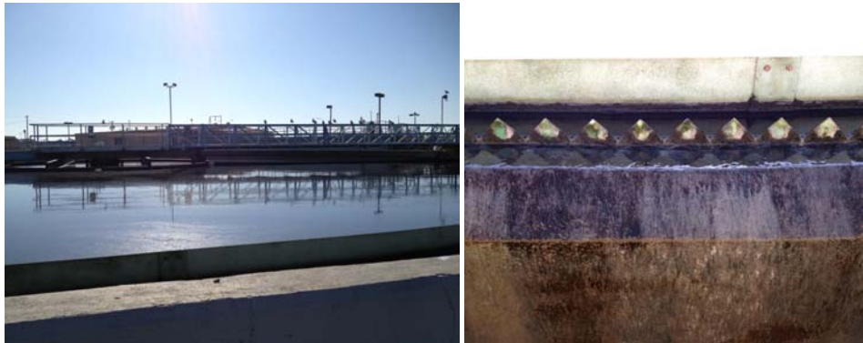
Figure 12: The secondary clarifier of the Marrero Wastewater Treatment Plant. The samples were pumped from the trough that the water spills into after flowing over the weir.
