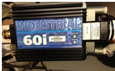
Figure 21: The 60i unit manufactured by HYDROFLOW USA utilizes the highest voltage of the models tested.
