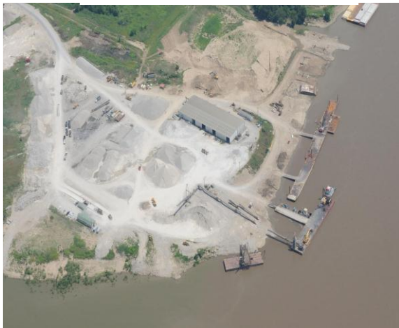
Figure 24 Fullen Dock Floating Barge
