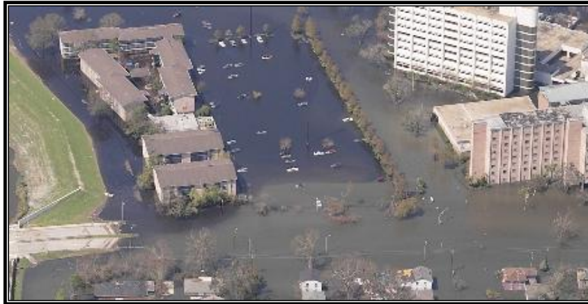
Major Flooding on UNO's campus and Leon C. Simon
