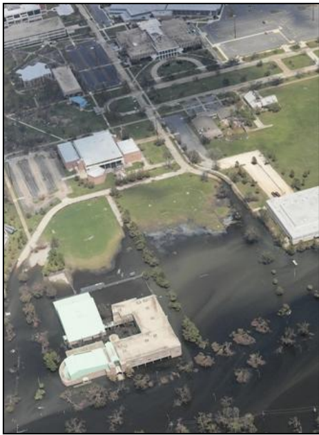
Flooding on UNO main campus from Hurricane Katrina
