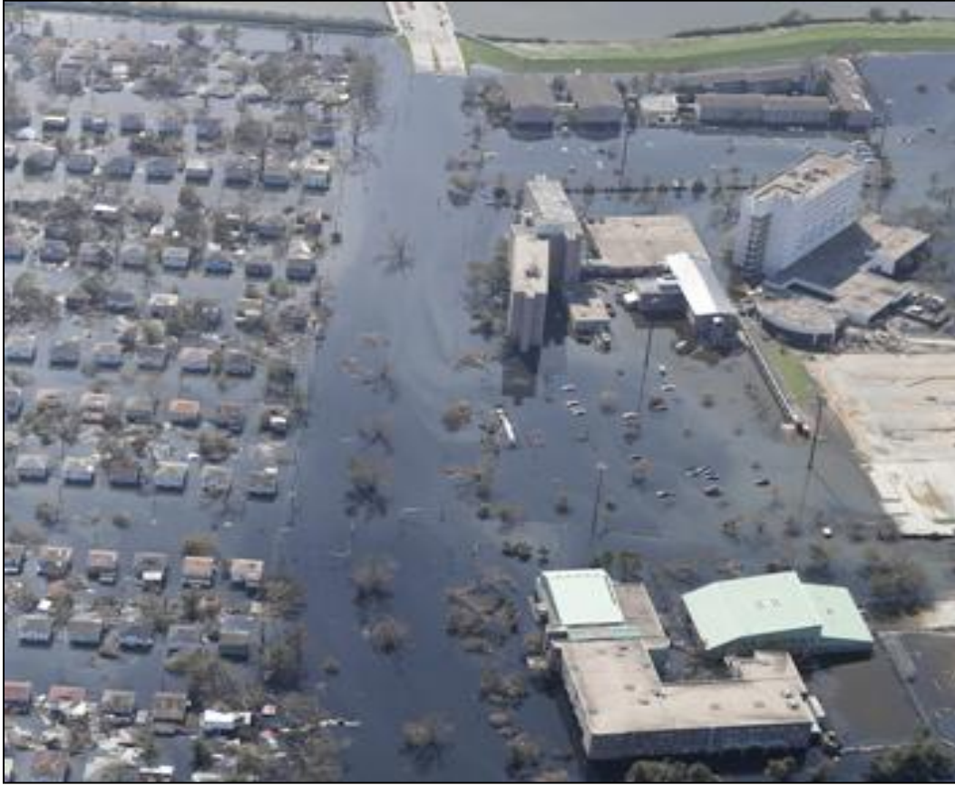
Flooding on Leon C. Simon Boulevard (southern boundary of campus)
