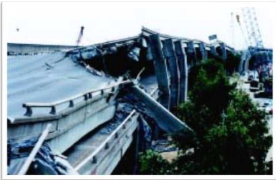
Figure 10 Cypress Freeway Damage
