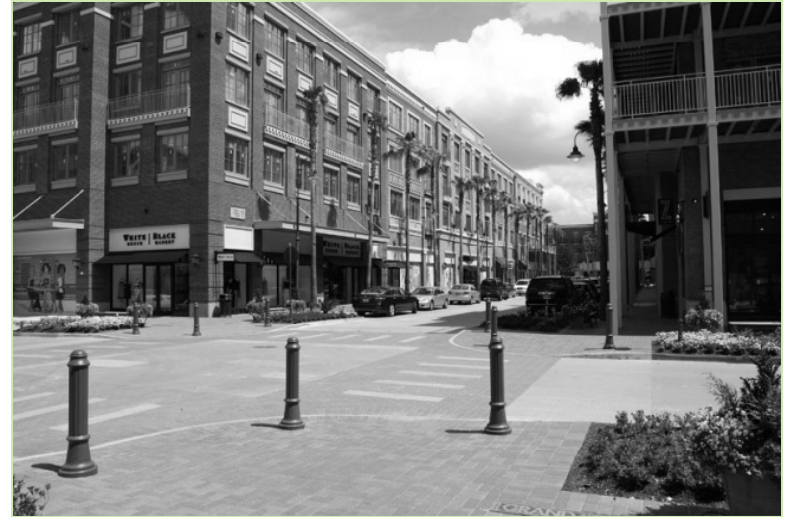
ABOVE: Perkins Rowe, Baton Rouge, Example of open air retail
