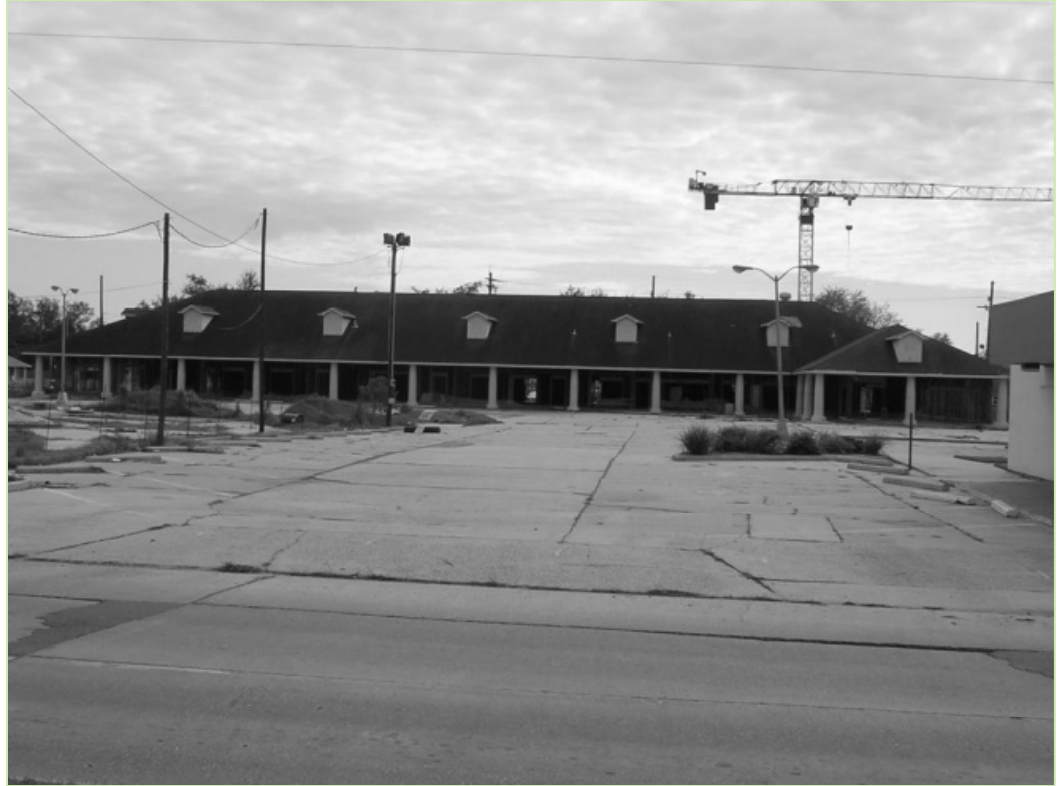
Above: A main structure of Lake Terrace Shopping Center
