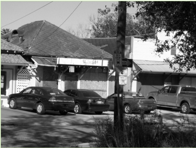
Above: Unoccupied and unrepaired buildings
