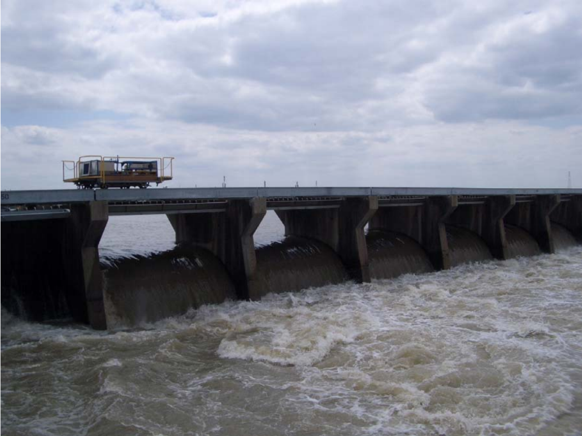
Figure 2.3 Photo showing flow through the open gates of the weir at the Bonnet Carré Spillway on April 15 th , 2008.
