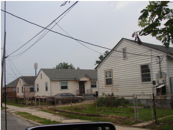
Figure 40. Barracks seen on Frenchmen Street Source: Author, October 2006
