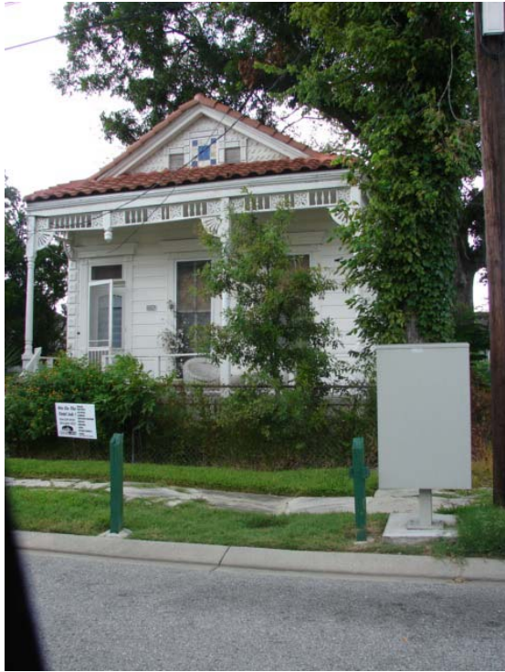
Figure 44. Arthur Richard House. Source: Author May 2006
