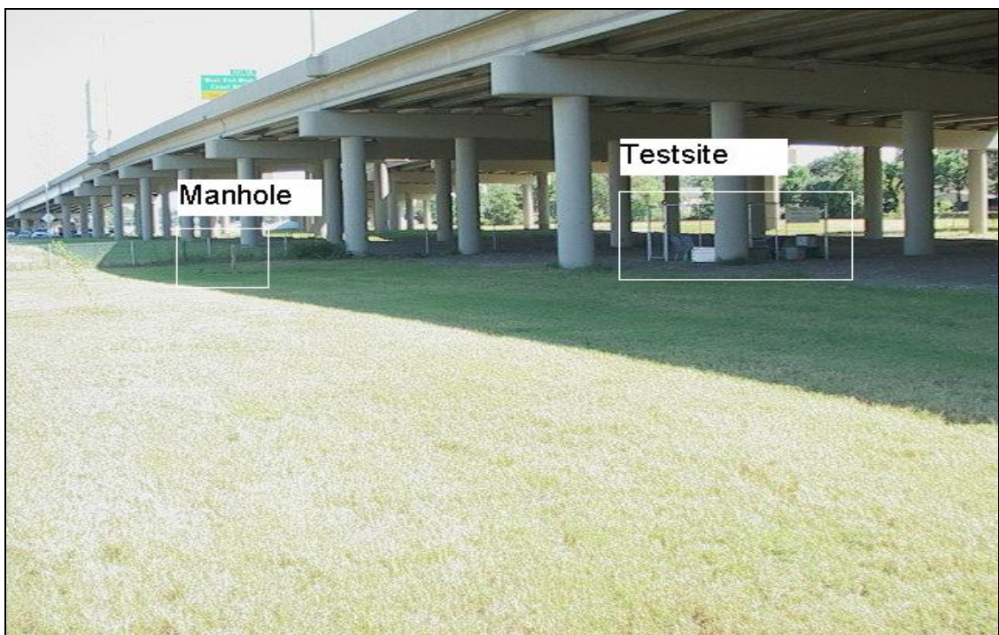
Figure 1: View of the Experimental Site and Manhole.
